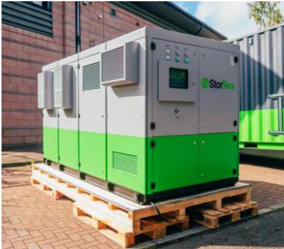
Figure 4 : BESS System Ready for Shipping
